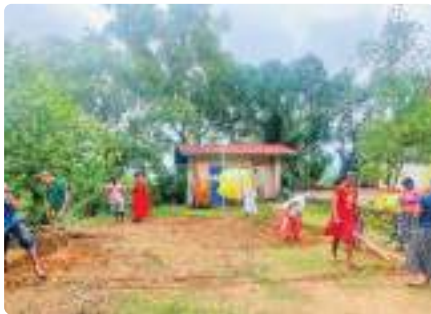
Two classrooms which are currently in the process of construction in Galle and Kurunegala.
