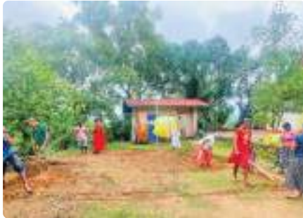
Two classrooms which are currently in the process of construction in Galle and Kurunegala.
